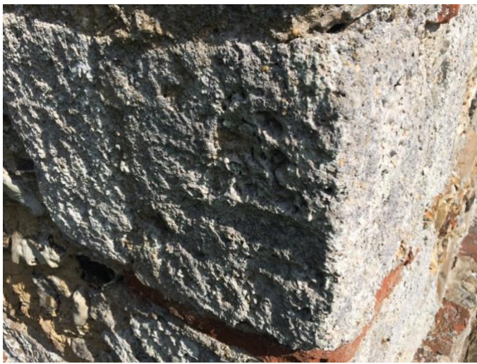
Tufa block quoin close up. Photo I Mercer 2017
