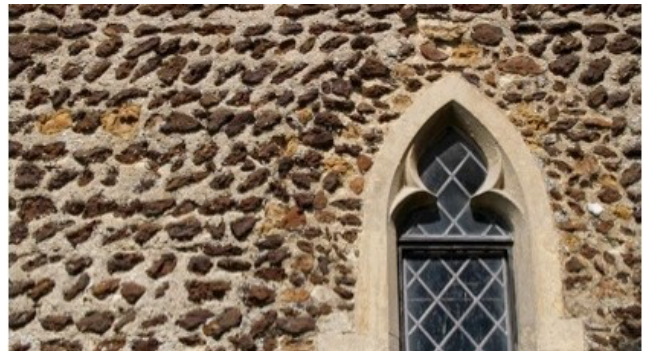
Great Bentley Church, an unusual example of a building constructed almost entirely from ferricrete. Photo: G. Lucy
