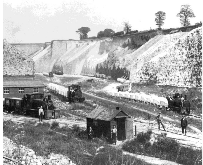
A Thurrock chalk quarry in operation in the 1920s. In this particular quarry the chalk was excavated from sloping faces and directed down channels into waiting railway wagons for transporting to the cement works.
